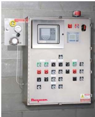
Flexicon offers NEMA 4 (shown with optional purge kit) and NEMA 7/9 (explosion proof) control panels.
